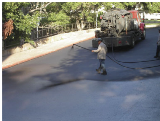
Spraying Parking Lot with Coal Tar Sealer
